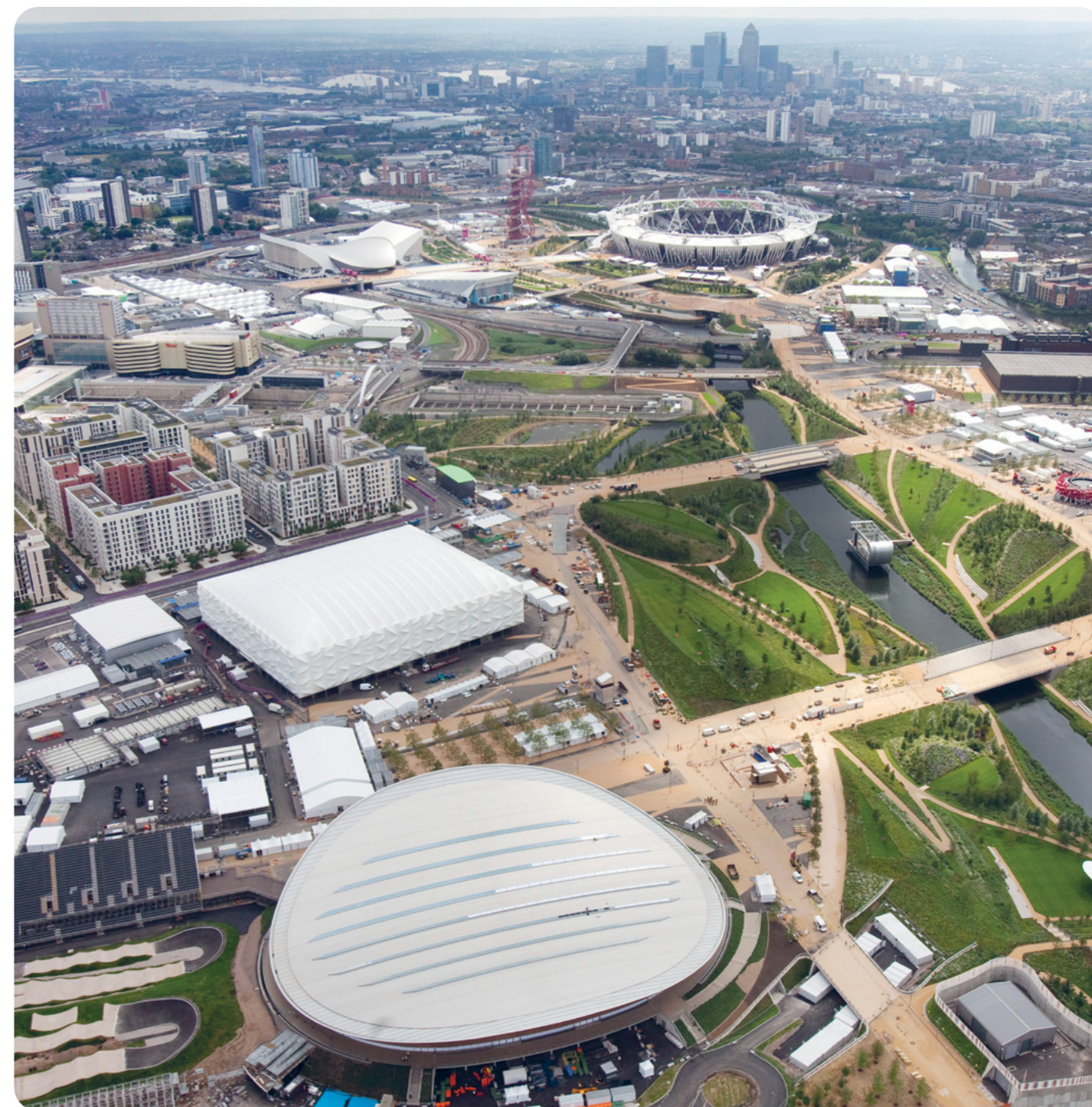
London 2012: aerial shot over Olympic Park.
